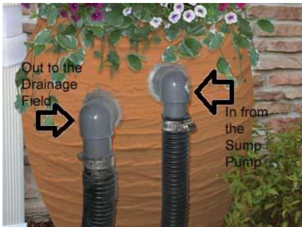
Collect sump pump water in a rain barrel to water plants and gardens. Drain before freeze-up.
